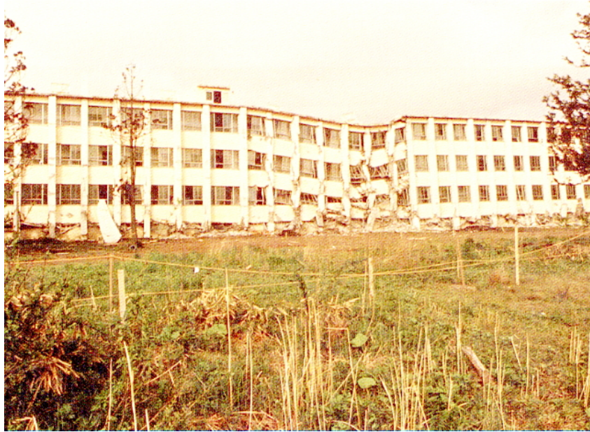
First Floor Damage in University Building
