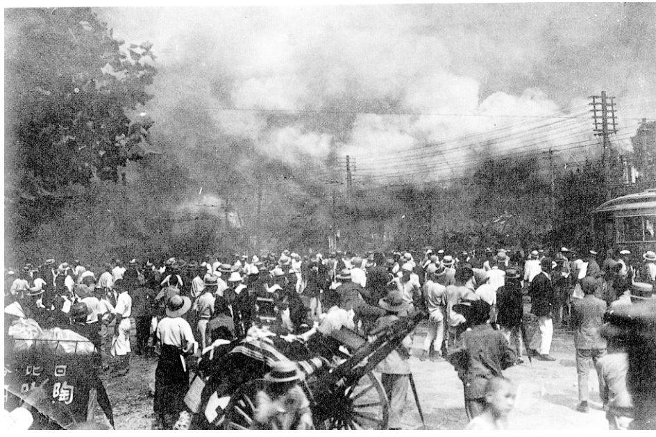
FIRE AFTER EARTHQUAKE
