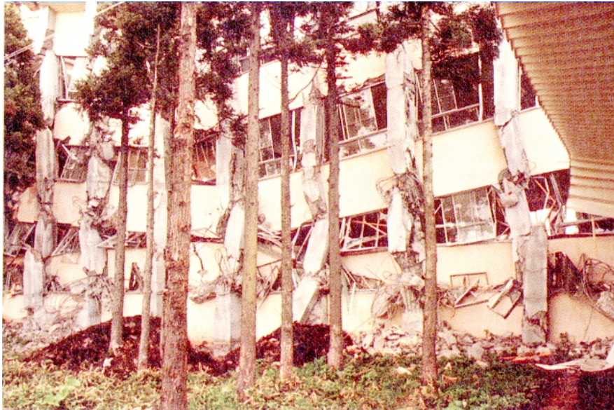
Share Failure of Short Colum
