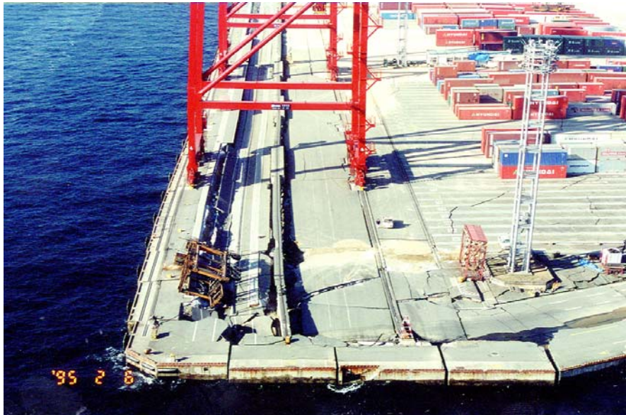
Side Slip of Pier
