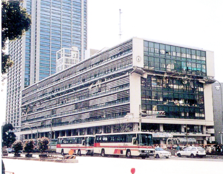
Collapse of Middle Floor
