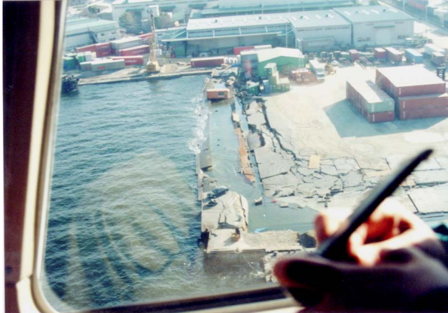
Side Slip of Pier
