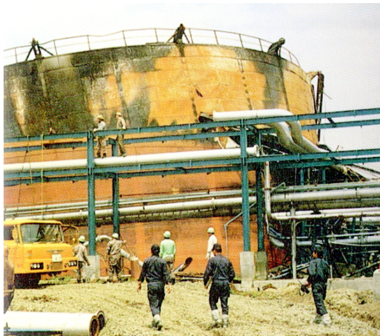
Floating Roof Petroleum Tank
