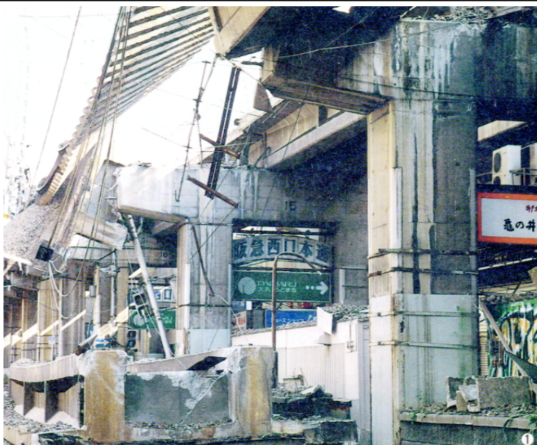
Rail Road Bridge
