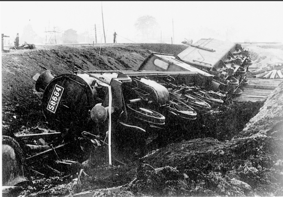
DERAIL OF S.L.TRAIN
