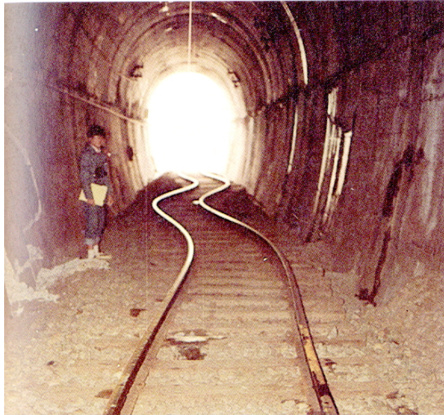
Railway Tunnel which Earthquake Fault passed
