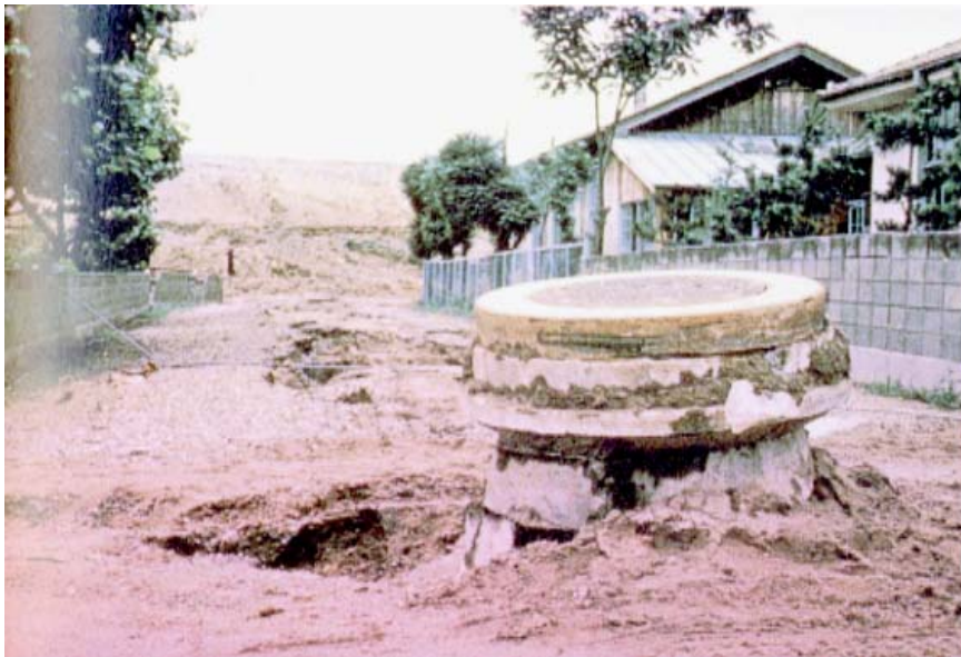
Up lifted Manhole by Liquefaction
