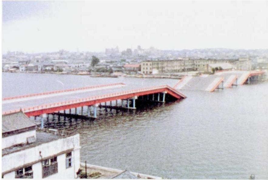
Fall down Simple Girder Bridge 伯野
