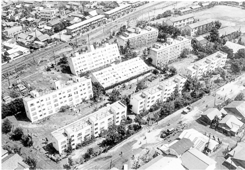
Leaned RC Structures by Liquefaction
